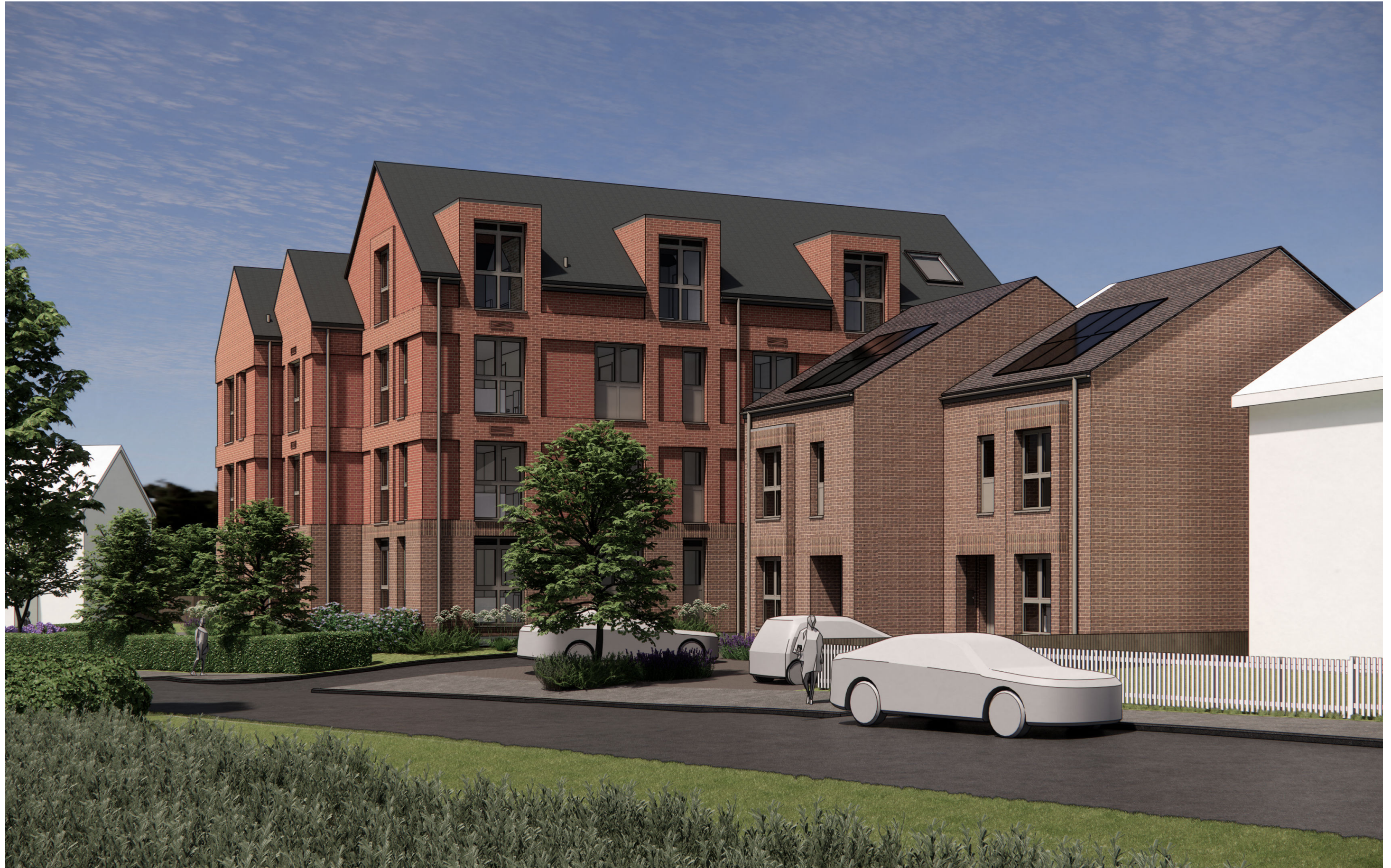
Dane Valley Road - Block B + C
