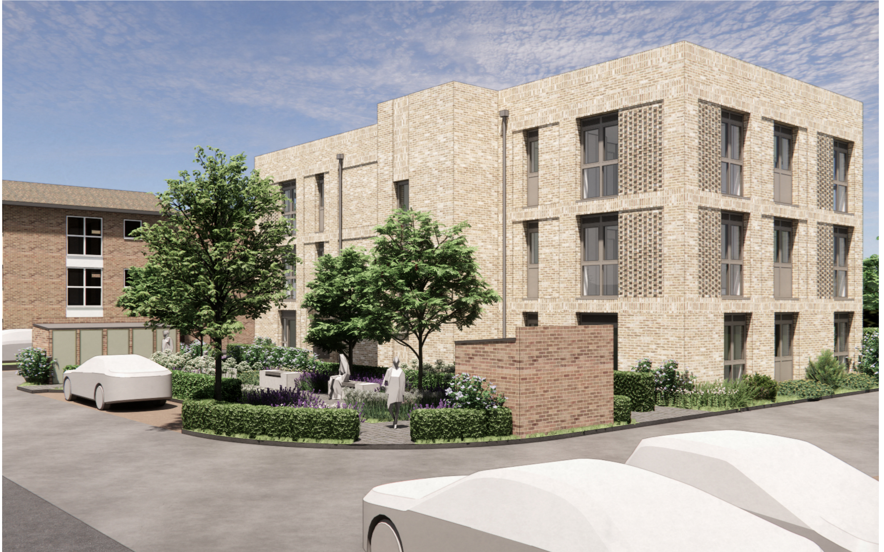
Clements Road - view from access road
