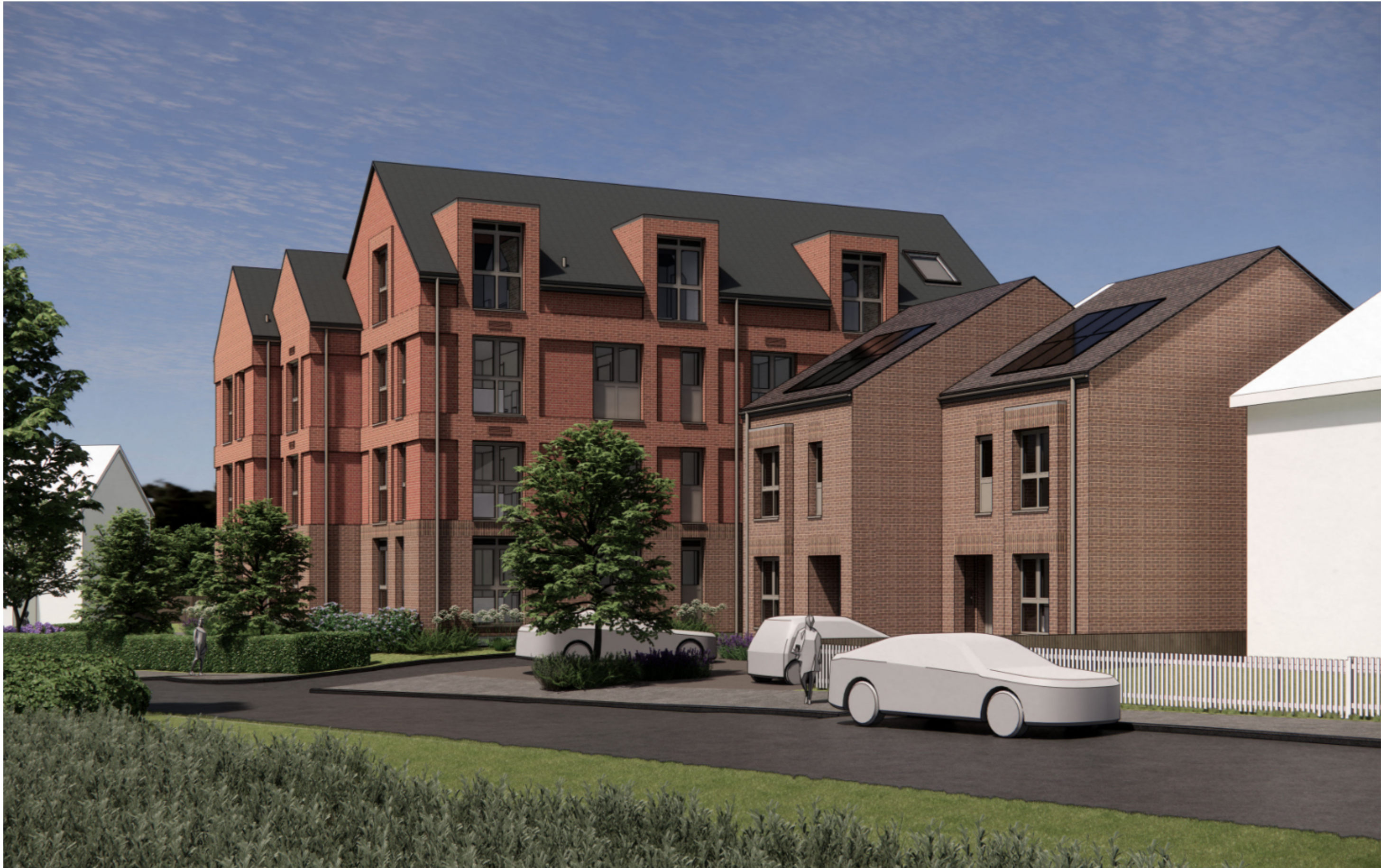
Dane Valley Road - Block B + C
